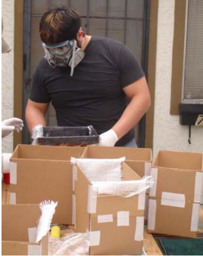
Figure 3.5. Fiberglass Construction Process. Cardboard frames were covered in fiberglass cloth and soaked in resin to create the rigid container.
